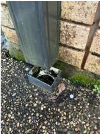
Few Downpipes damaged/cracked/dismounted or not properly connected to stormwater system- Recommend engaging a Plumber to repair & avoid the risk of foundation movement & other moisture related issues.
