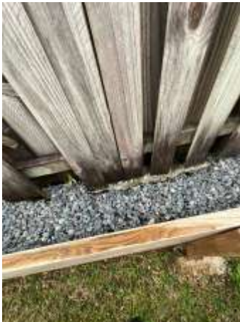
Leaning fences to parts - recommend engaging a Builder or Fencer to rectify to prevent further deterioration.
