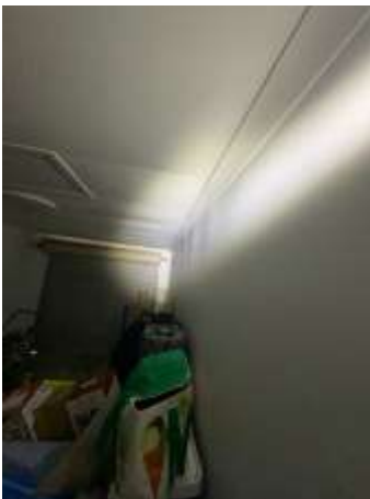
Sagging and Creasing visible on ceiling plasterboards, Recommend repair by engaging a licensed Plasterer.
